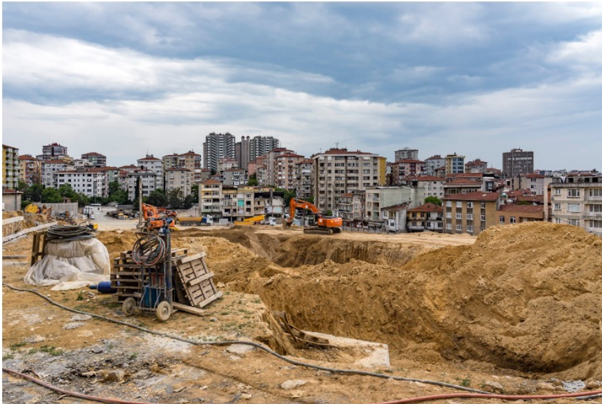
Figure 4.9 Kadikoy-Fikirtepe Construction Area in 2019 (Murat Germen)
